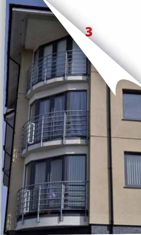
28 flats and commercial units were built on the site of the former Vivian Park Hotel, Aberavon, Port Talbot
